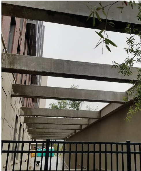
Before (left) and after: Upon seeing the beautiful direct-applied stucco on its Chevy Chase Lake garage ramp retaining wall, the developer, EYA, also requested that stucco be added to the structure's raw concrete horizontal support beams.
