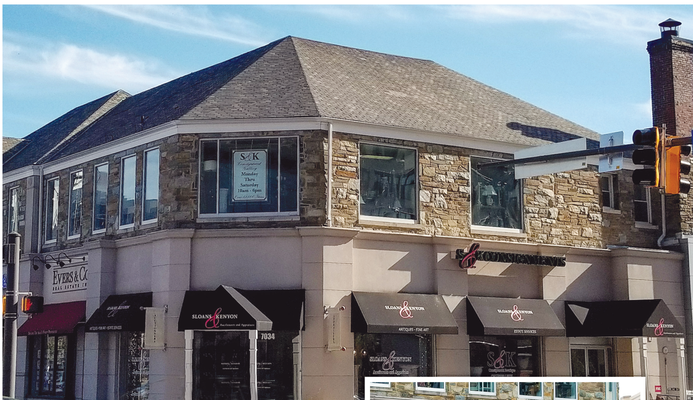
Above & right: Glaser Construction LLC applied synthetic stucco to this commercial storefront in Bethesda, Maryland.
