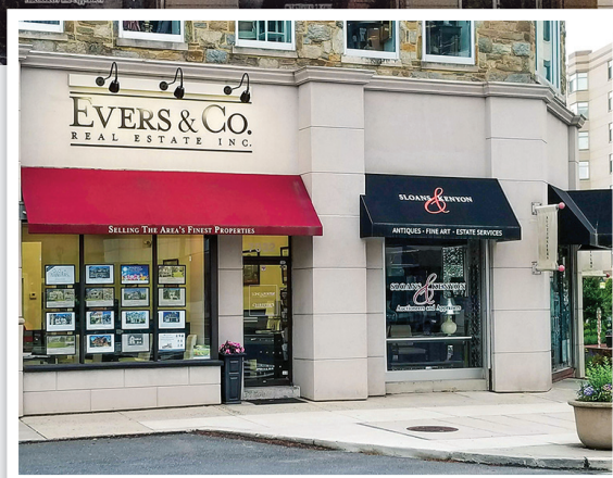
Above & right: Glaser Construction LLC applied synthetic stucco to this commercial storefront in Bethesda, Maryland.
